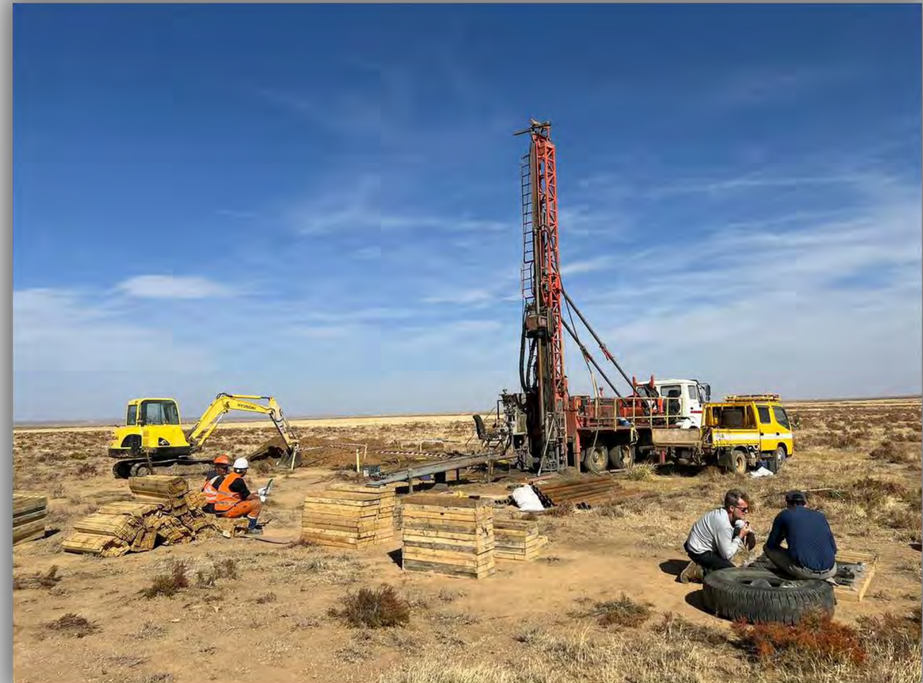
Diamond core drilling at UNDH-02
